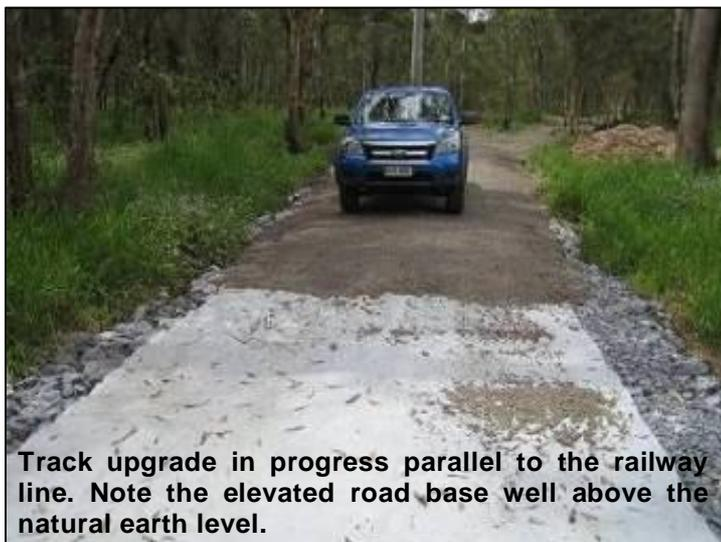
Track upgrade in progress parallel to the railway line. Note the elevated road base well above the natural earth level.
