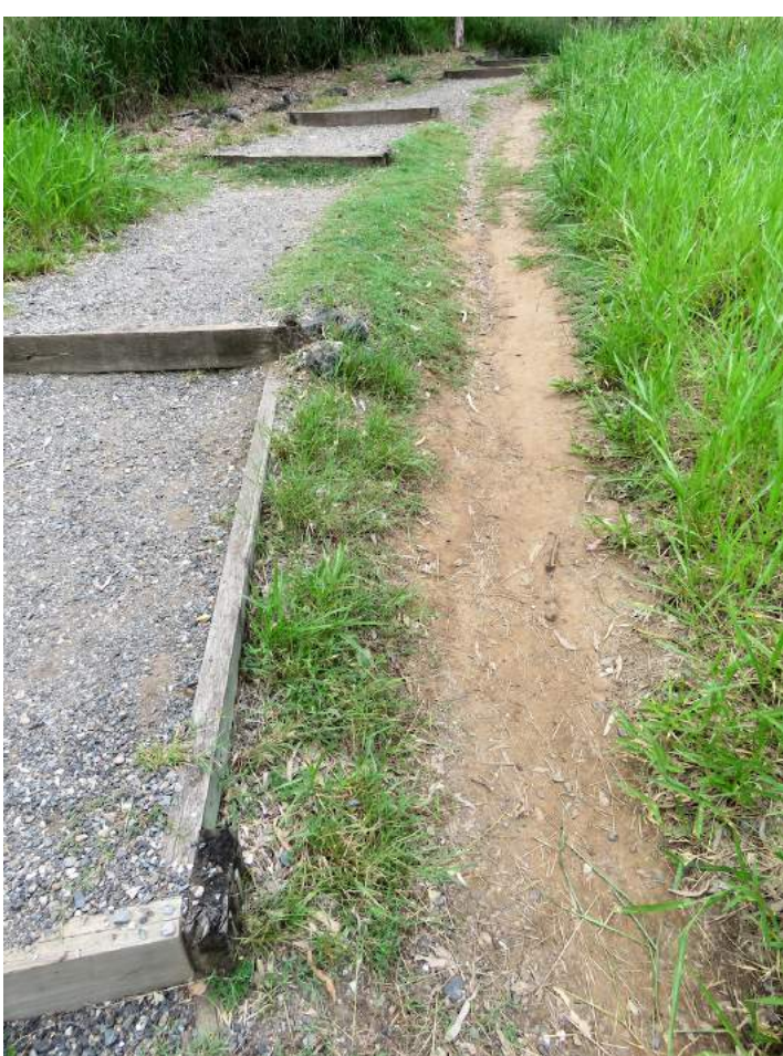
Erosion caused by bikes avoiding the steps on Coucal Trail (Photo © Vaughan Kippers 10:29, 17 April, 2021)
